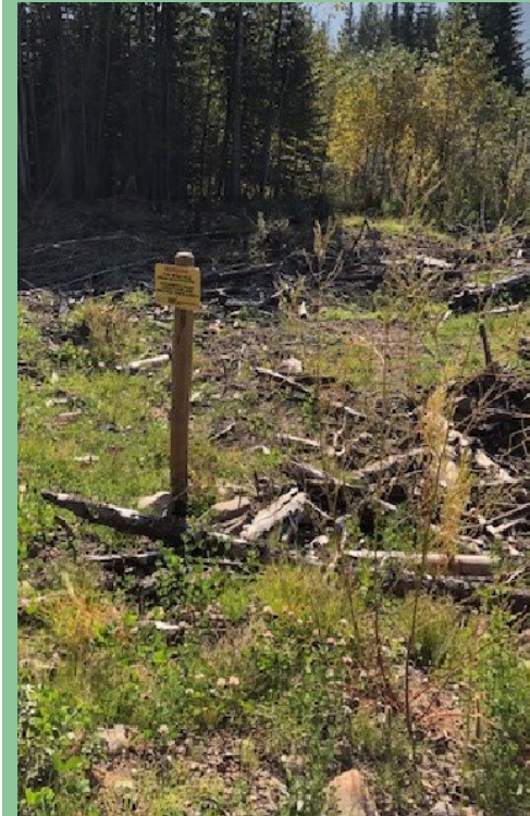
At the Canfor Chetwynd operation a road has been deactivated and vehicle access is no longer possible. A notification sign has been posted making road users aware that the road has been deactivated.
